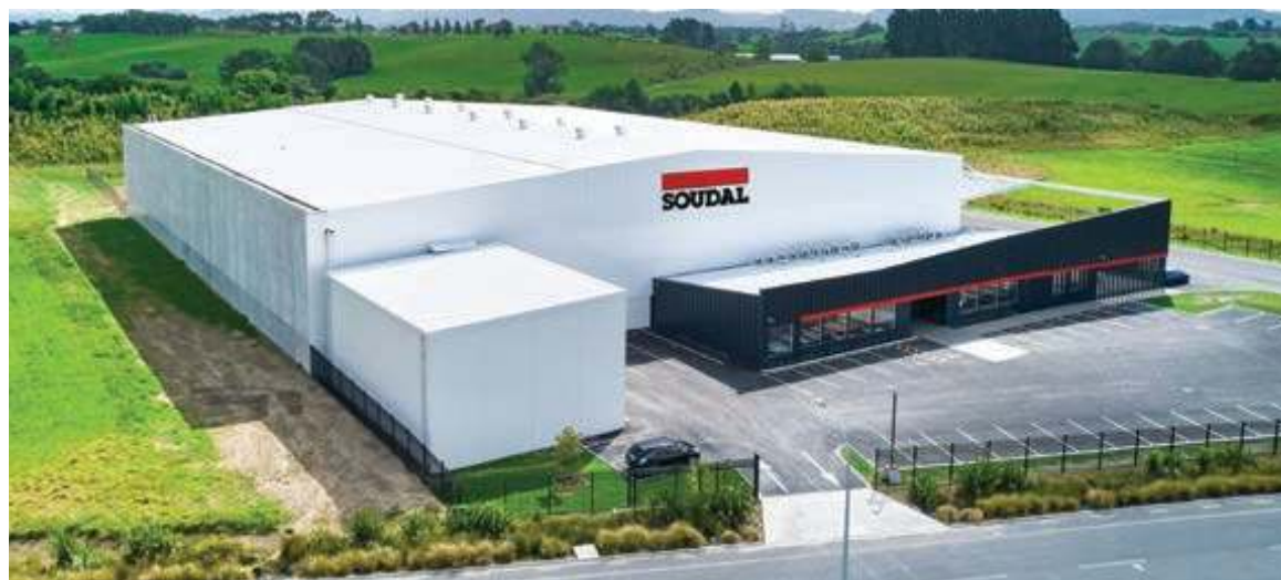
New distribution centre with office building • New-Zealand
